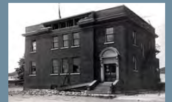
Damage to School and Post Office from Earthquake | Courtenay & District Museum, 972.54.2 and 2004.10.1
